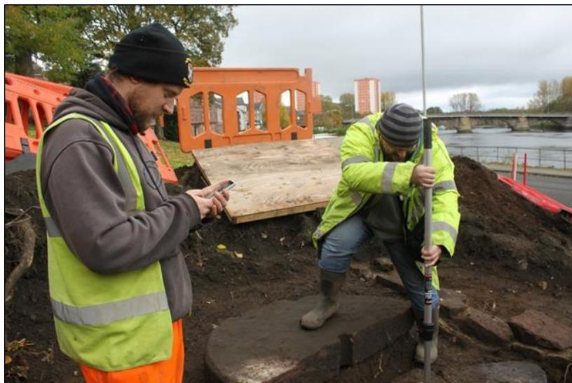
Using Camera mounted on pole to record the bottom of the well with mobile for DSLR remote.
